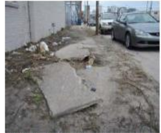
Sidewalks are missing or damaged on Tulane Avenue at S Dorgenois St
