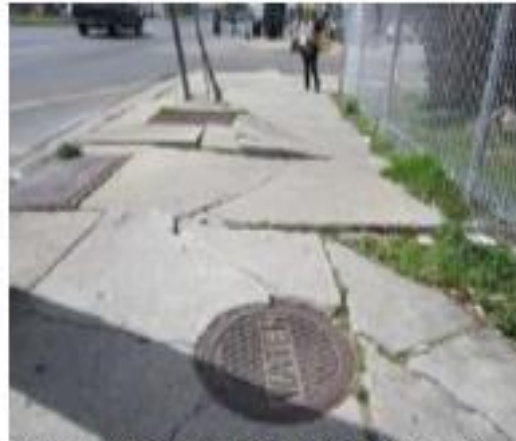
Severe trip hazards on South Broad Street at Tulane Avenue
