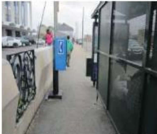
Narrow pedestrian access zone on South Broad Street at Canal St impedes accessibility
