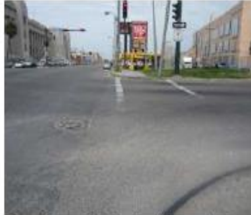
Crosswalks are faded and missing; curb and median lack ADA ramps at Tulane Avenue and South Broad Street
